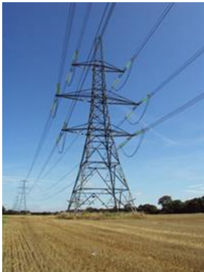
Figure 3.2 – 400kV Steel Lattice Angle Pylon
