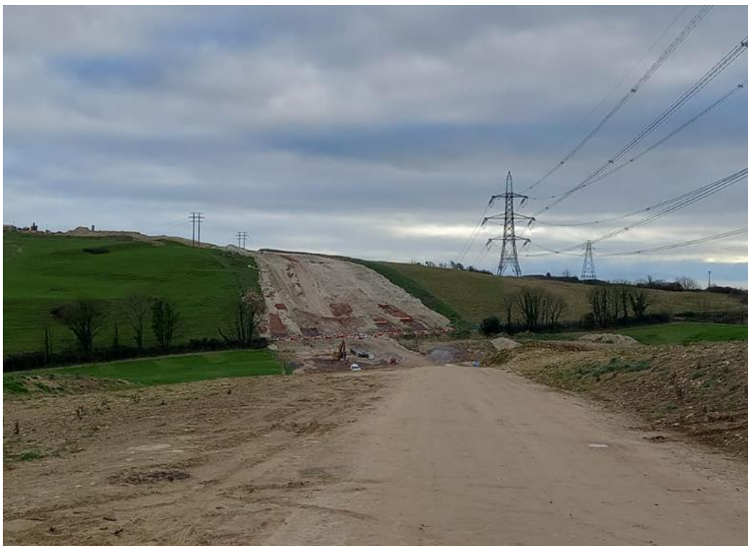
Figure 3.4 – 400kV underground cable swathes
