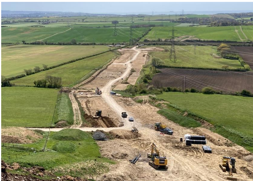
Figure 3.3 – 400kV underground cable swathes
