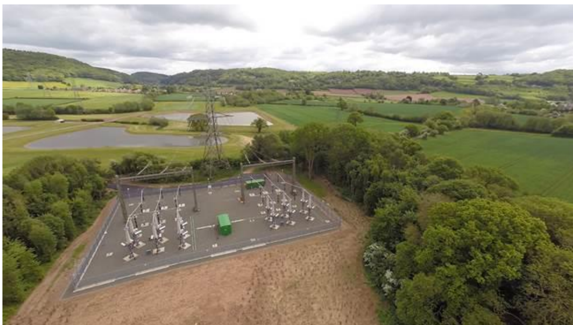
Figure 3.5 – 400kV Cable Sealing End Platform
